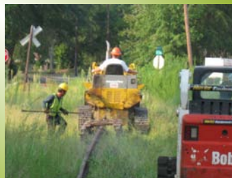
Workers Removing Trails
