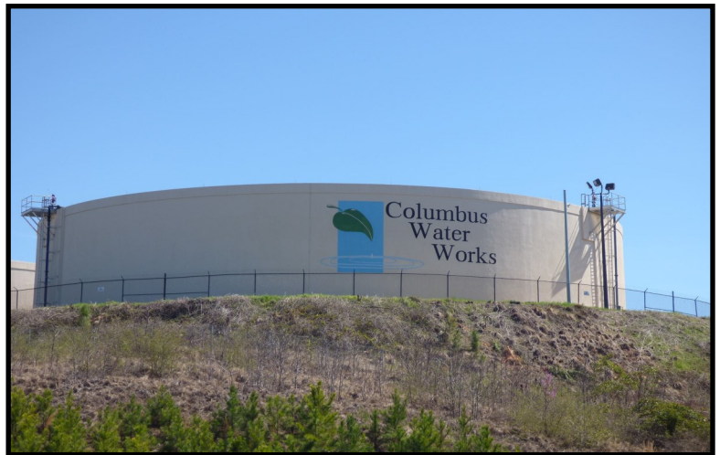
Columbus Water Works Treatment Facility
