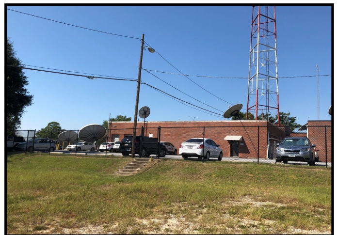
WRBL Station and Broadcast Tower
