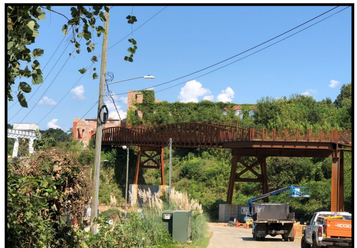
River Walk Bridge Expansion
