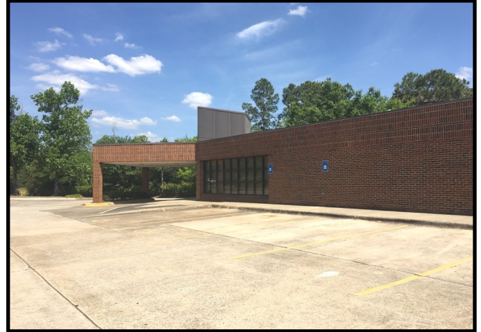
Vacant Medical Office Building
