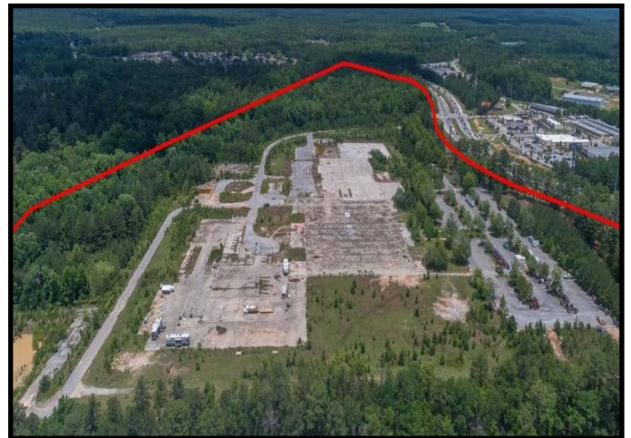
Swift Spinning Mills Site Aerial
