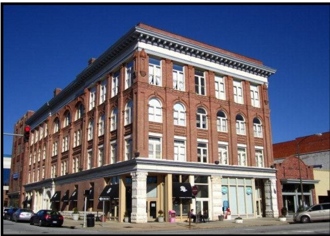
Traditional storefronts with living space above
