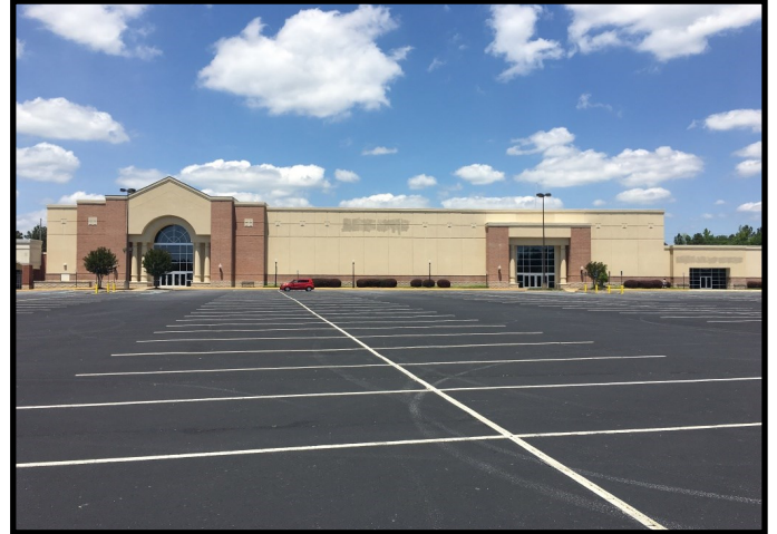
Vacant Sears Building
