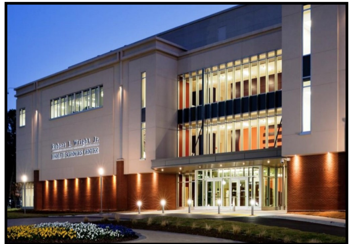
Classrooms at Columbus Tech
