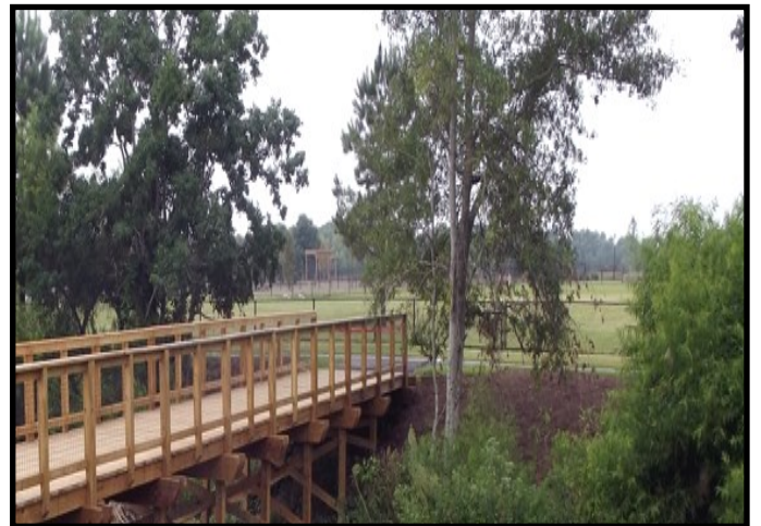
Oxbow Meadows Support Facility
