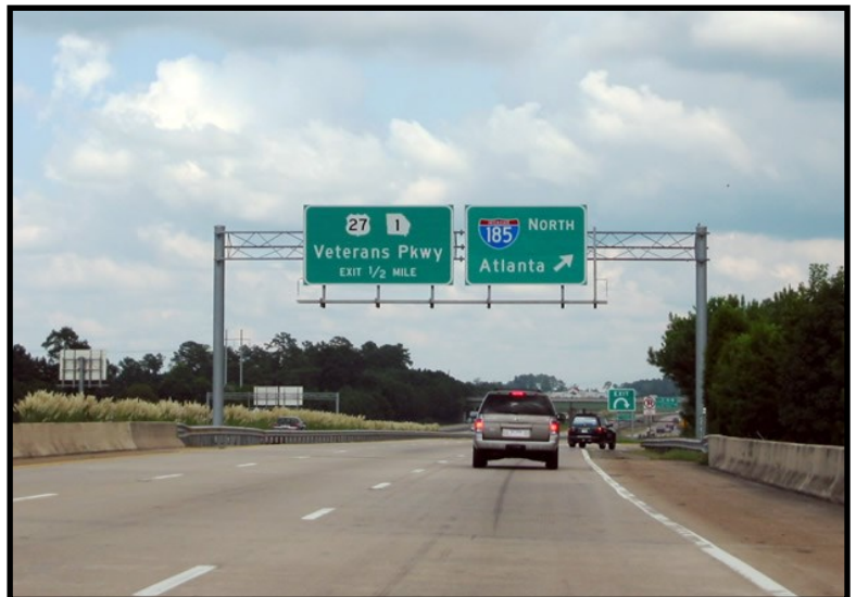
US 80 and Interstate 185 Interchange
