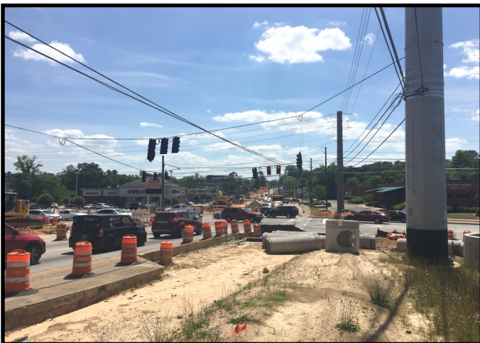
Talbotton Road Widening Project
