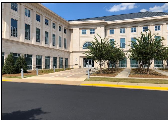
Muscogee County School District Admin. Building
