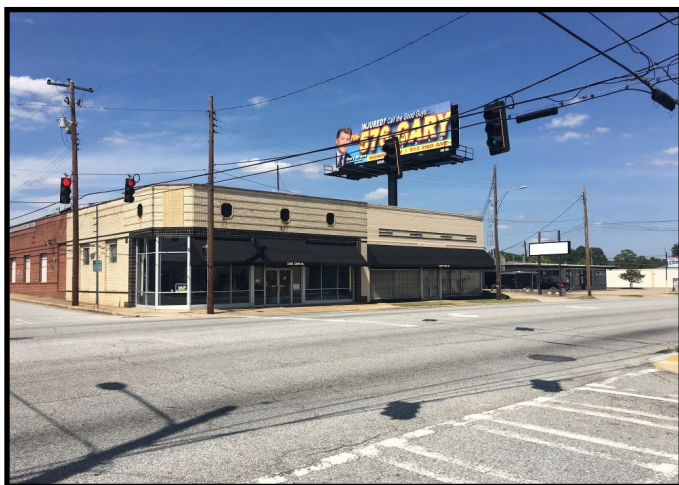
Vacant Storefront along 13th Street
