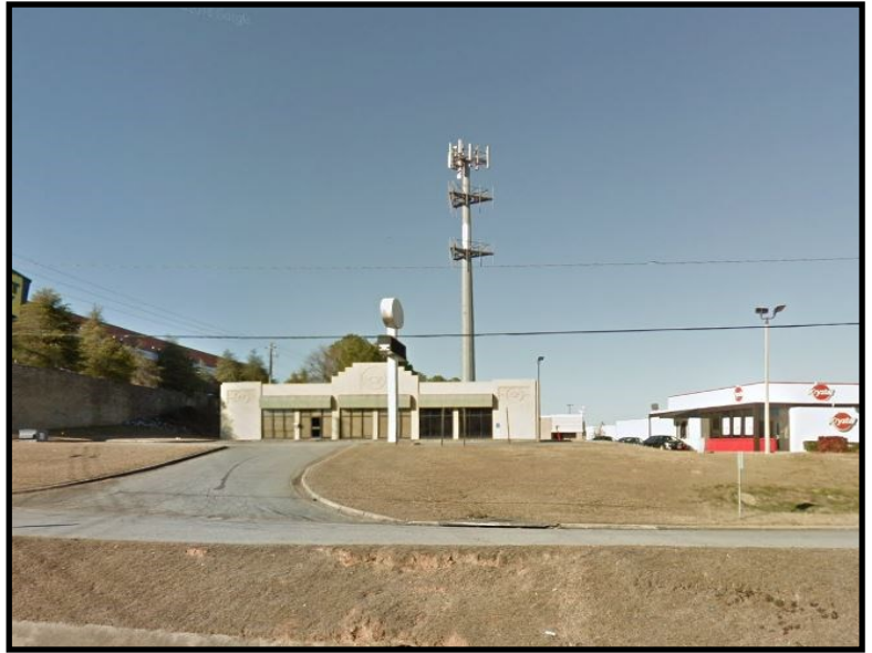
Cell Phone Tower along Manchester Expressway
