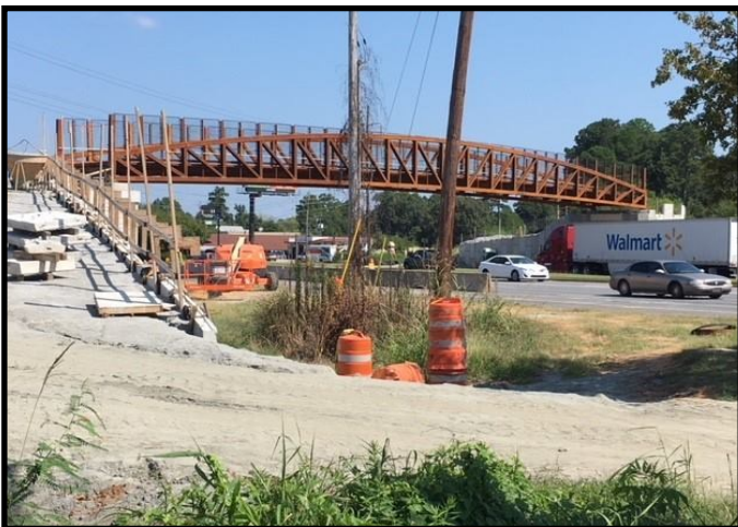
Follow Me Trail Bridge being installed
