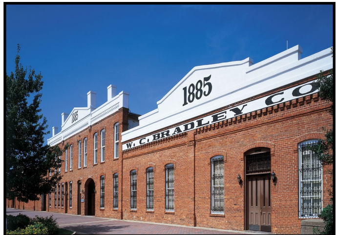
W.C. Bradley Co. Building
