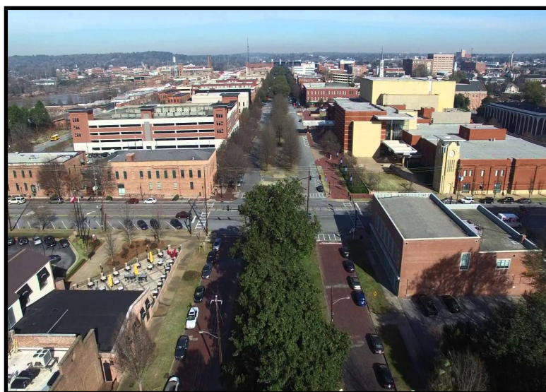
Broadway Facing North
