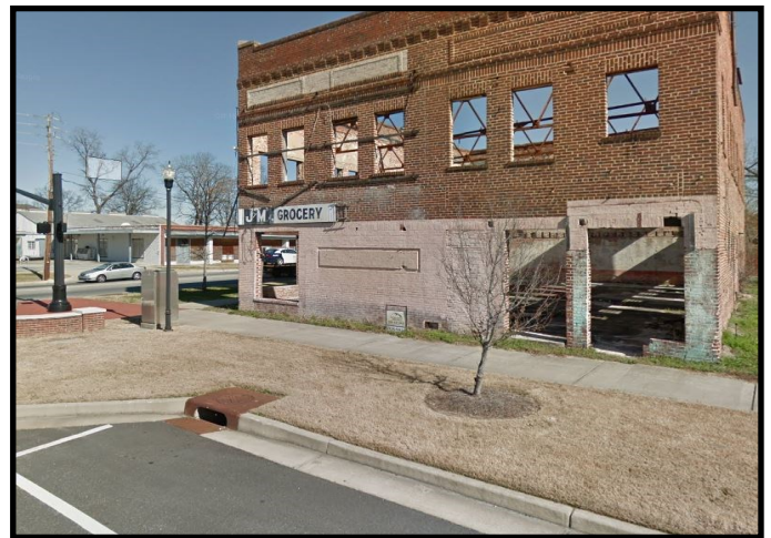
Dilapidated building along 6th Avenue
