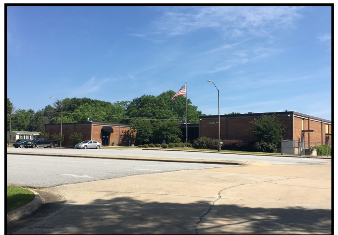
Georgia Power Office on Gentian Road
