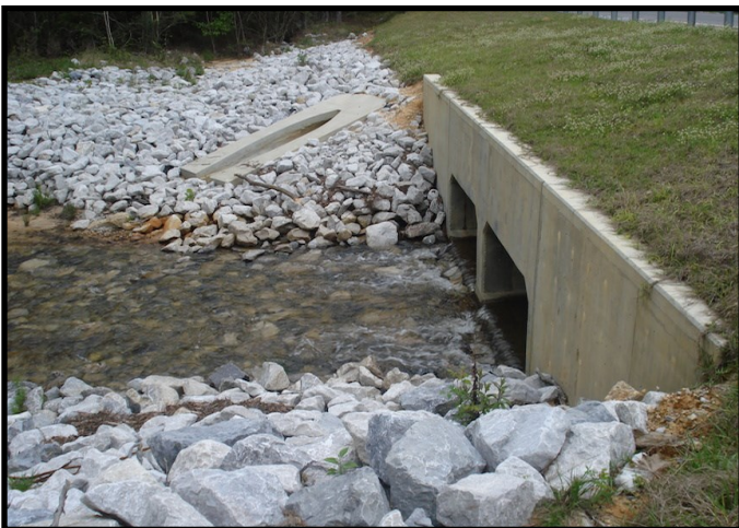
Lindsey Creek passing through a culvert
