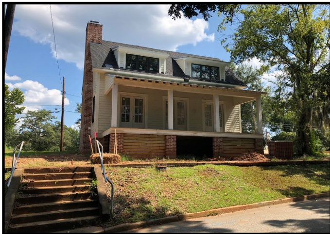
New single family housing under construction
